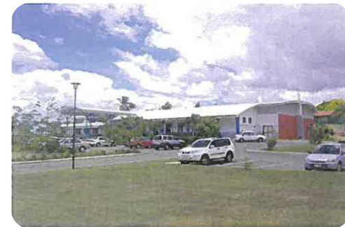
Loans from the Capital Fund have enabled the construction of a number of churches including the Creek Road Presbyterian Church pictured above.
